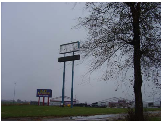
Broken sign on south side of vacant hotel property.
