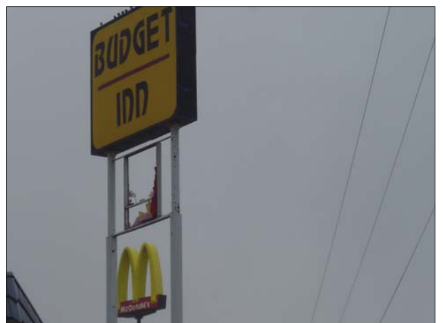
Broken sign on east side of South Route 45.
