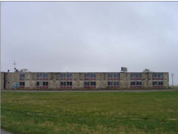
Rear of vacant hotel.
