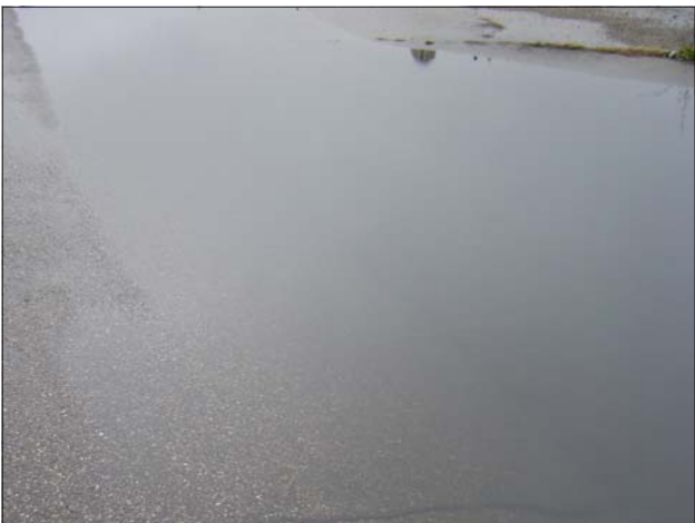
Standing water at entrance to vacant hotel on shoulder of Paradise Road.
