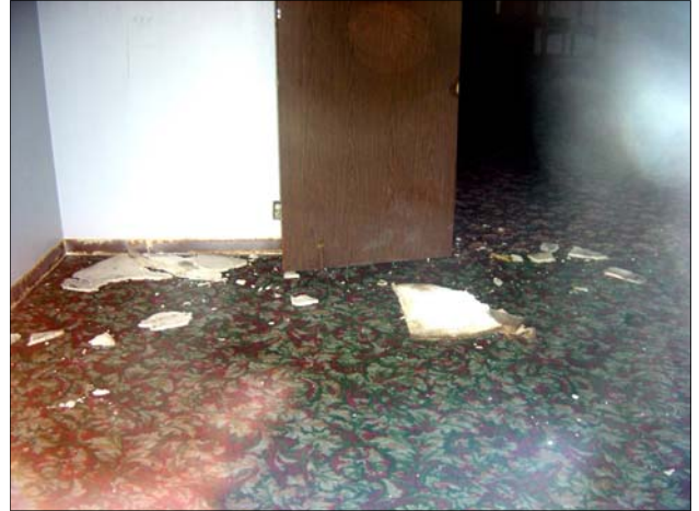
Falling ceiling tiles on floor of hallway in vacant hotel. Note the mold on the base of the walls.
