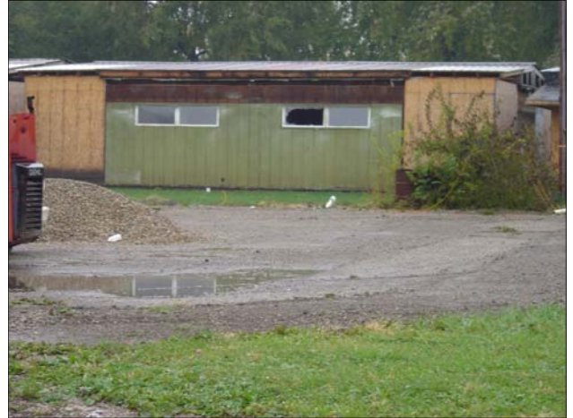
Dilapidated two-family apartment building. Note deteriorated pavement and broken windows.
